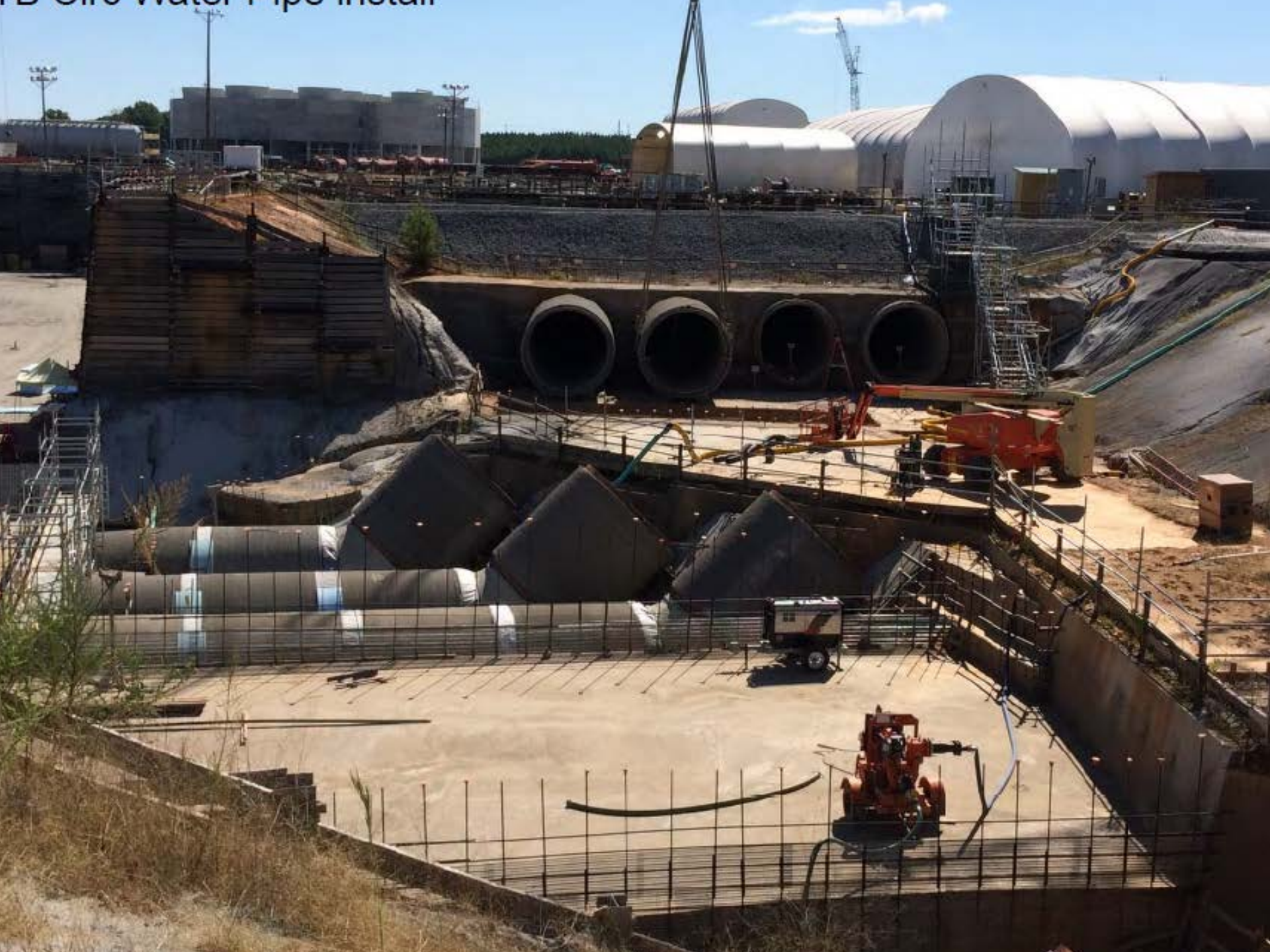
Drinking Water Pipe Installation
